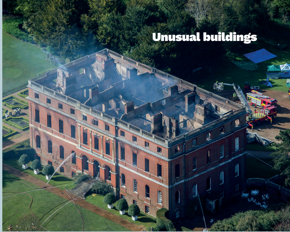
◻ The 2015 Clandon Park fire, which damaged all but one room, was caused by an electrical fault
