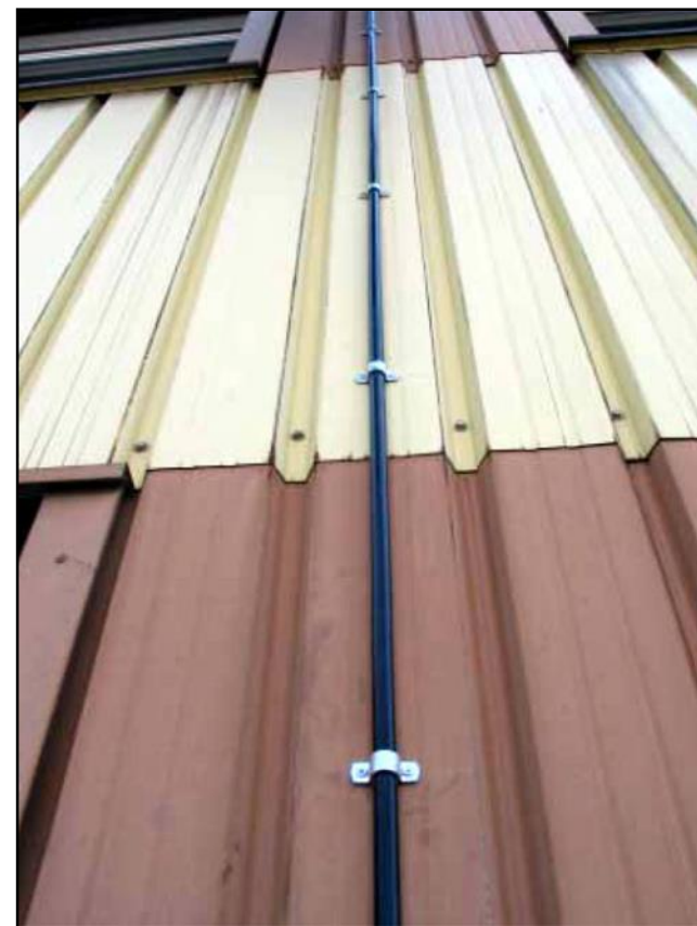
HVI® installation on the facade
