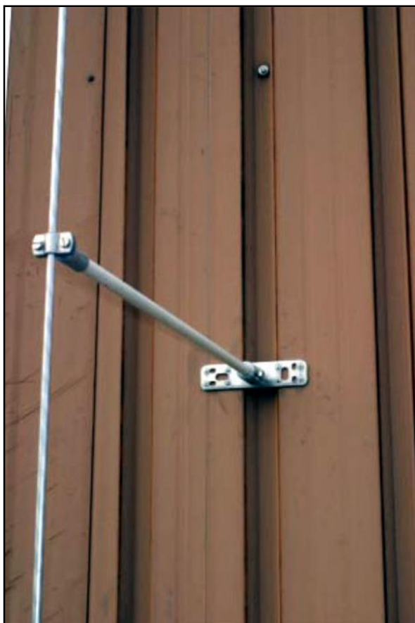
Installation of the distance holder
